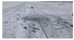
The aerator was installed on January 12<sup>th</sup> on the Maple Bay end of the lake. This aerator ensures that the oxygen remains at a safe level and the board tests the oxygen level throughout the winter.
